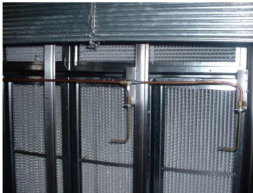
Pressure Transmitter Locations Figure 6
